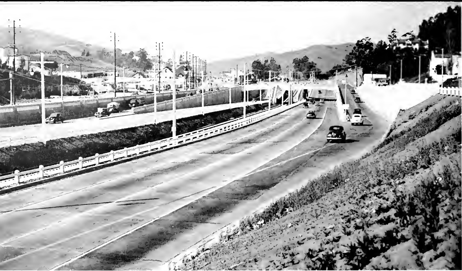
New section of Cahuenga Pass looking north toward Barham overpass, showing two 4-lane highways separated by railroad tracks with ramps to service roads
